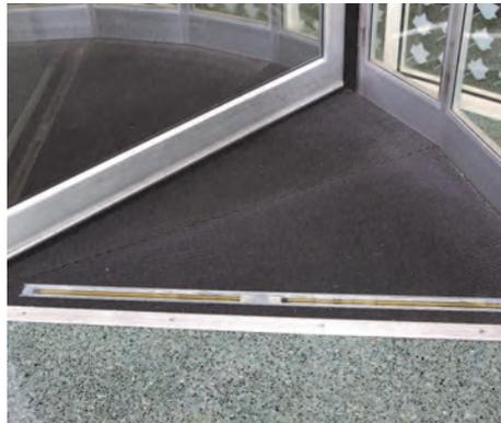
The door's object detection technology (in floor and overhead) senses undesirable and dangerous objects and prevents reentry, shutting the door down and sounding an alarm if something is detected.
